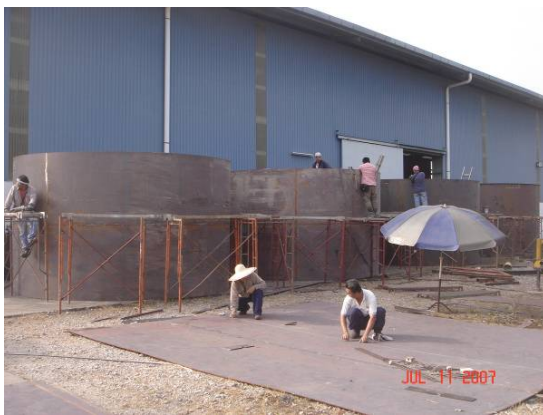
Cyclone casing and down-chute
