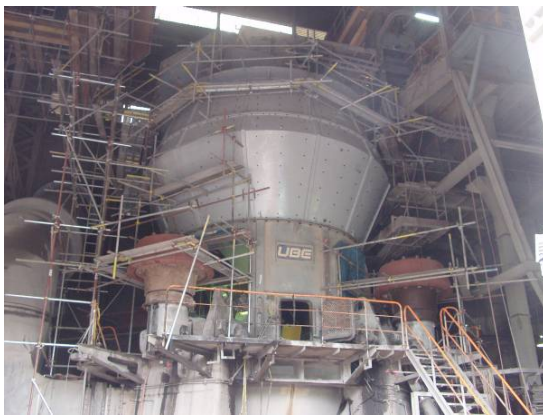
Raw Mill Classifier erection and Rotor alignment
