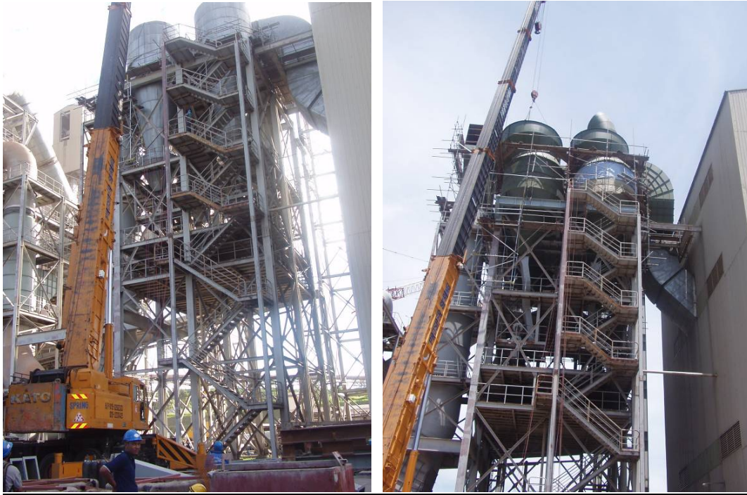
Raw Mill Cyclone erection
