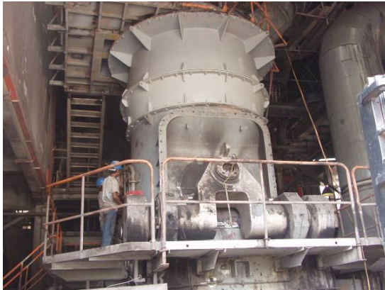
Coal Mill Classifier erection
