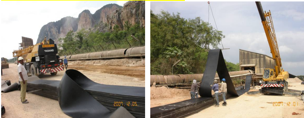
Our installation team at CIMA, Perlis.
